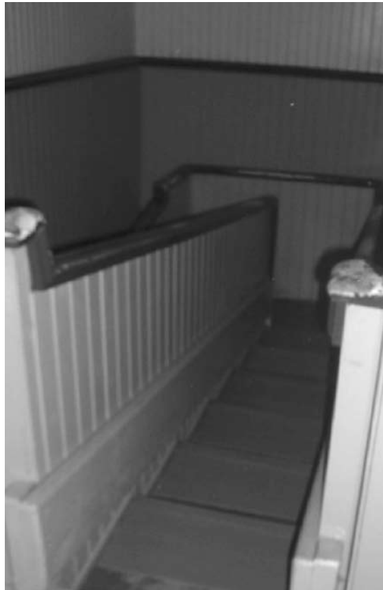
Staircase to nowhere
