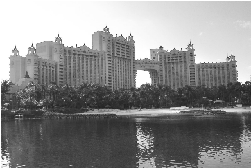
Atlantis Hotel – Royal Towers
